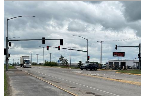
The intersection of River Drive and 38 th Street North is signalized.
